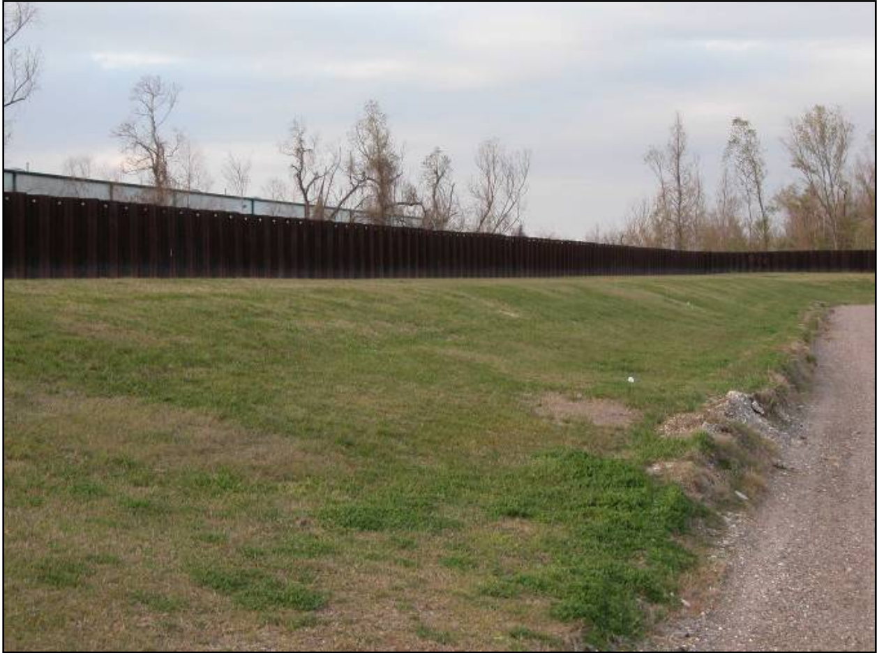
Figure 7. Typical sheet-pile I-wall.
