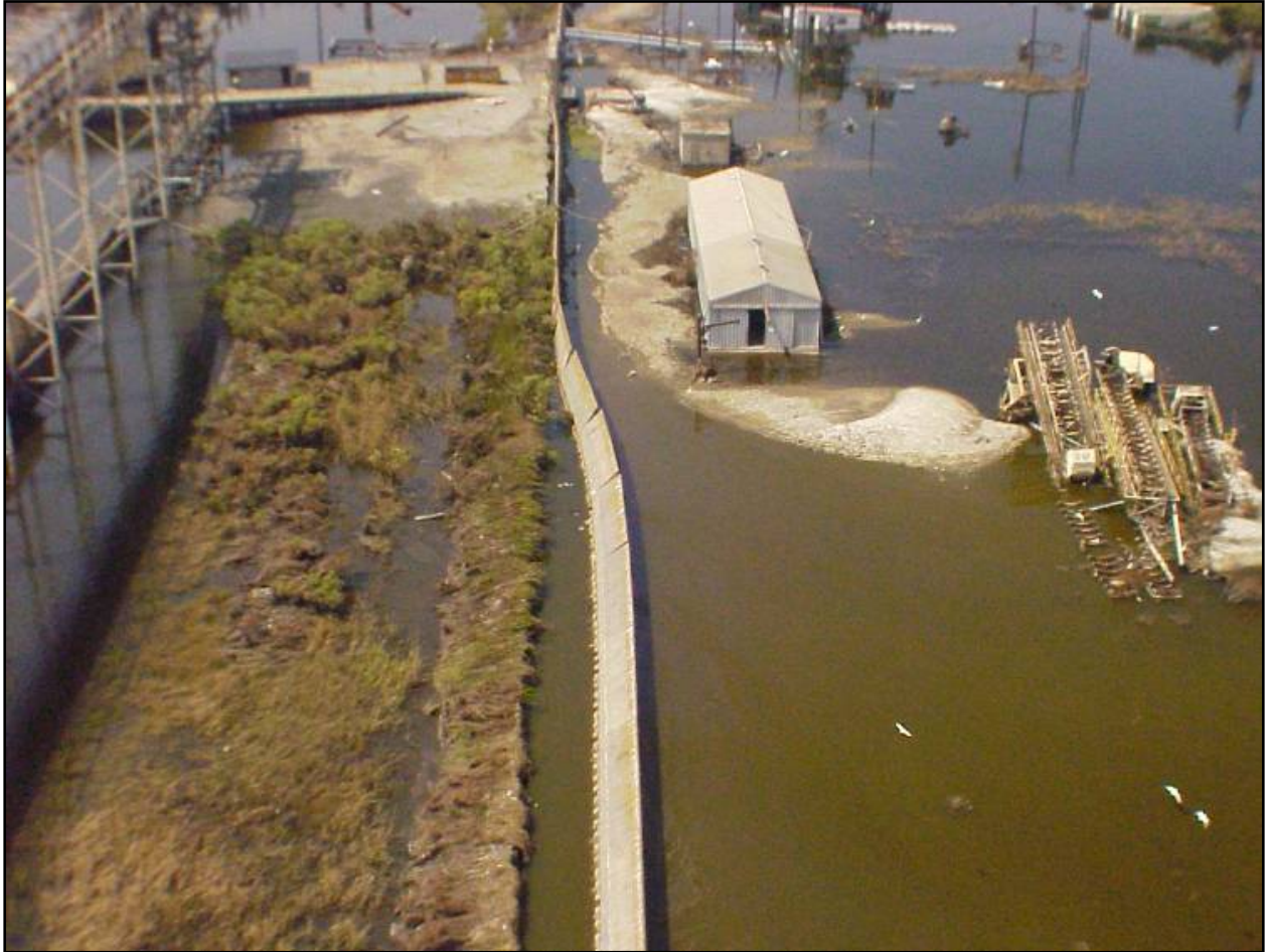
Figure 11. Katrina damaged I-wall.
